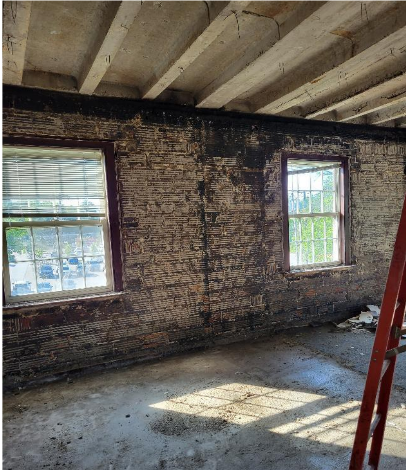
Ext. Wall After AeroBarrier
