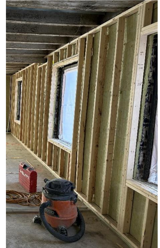
Wood Studs Installed
