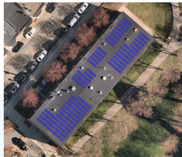
First Solar Project East Boston YMCA
