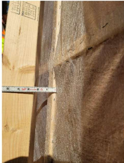
Figure 5. Location and spacing of netting staples
