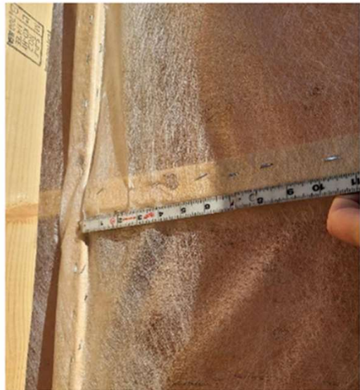
Figure 4. Location and spacing of netting staples
