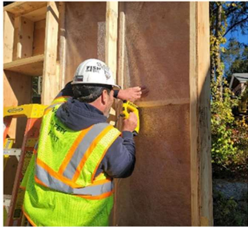
Figure 3. Stapling insulation netting
