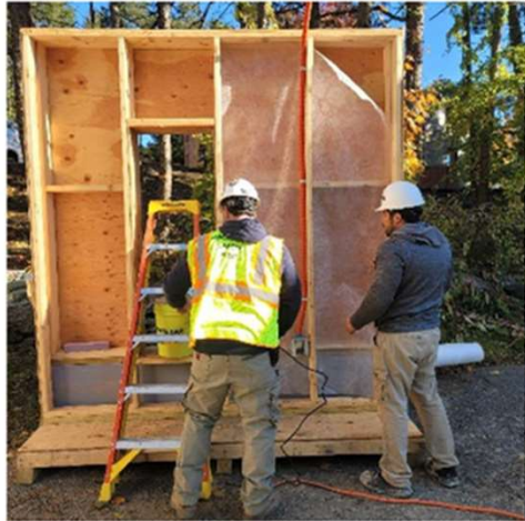
Figure 2. Cellulose insulation netting install
