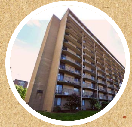
Existing Building Decarbonization
