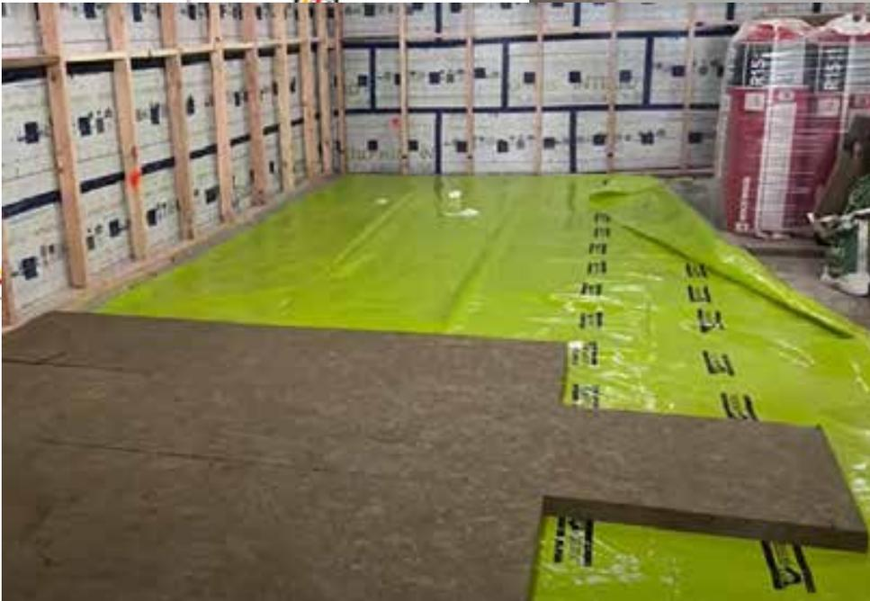
Floor airbarrier – PE sheet over existing concrete + 2.5" Rockboard 110 (R9)
