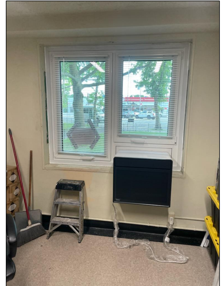
New triple pane casement window with heat pump sleeve, from Intus Windows
