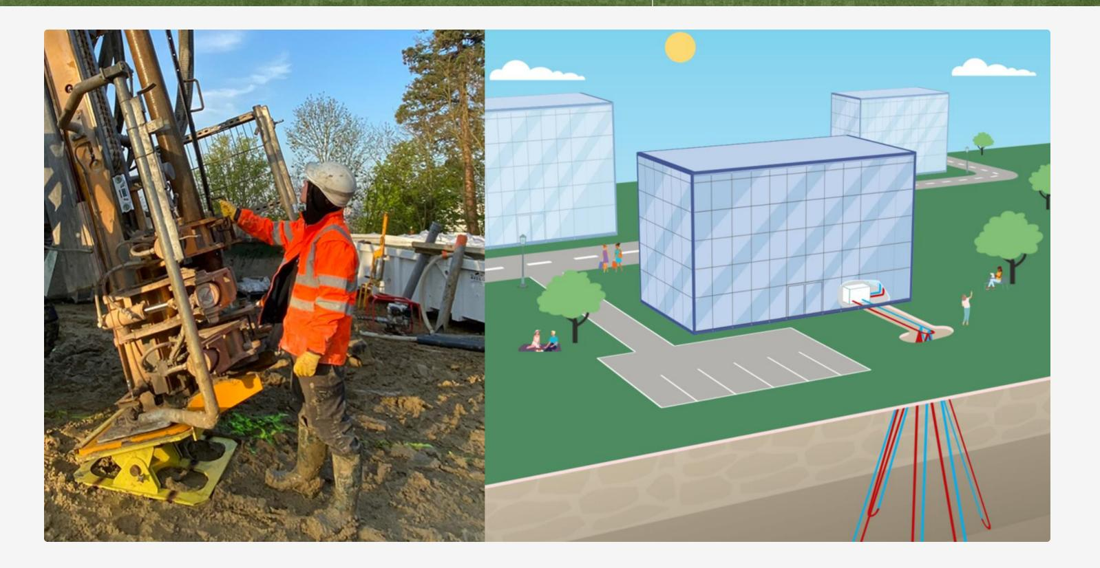
Angled drilling can increase the capacity of a system by up to 30% by decreasing the amount of surface space needed
