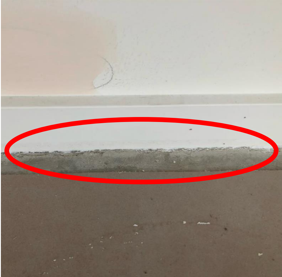
AeroBarrier Sealant at Bottom of Party Wall
