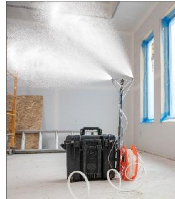
Computer Controlled Sealing Station Spraying Sealant
