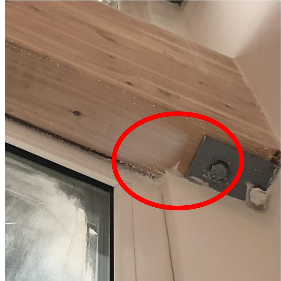
AeroBarrier Sealant at Exterior Wall
