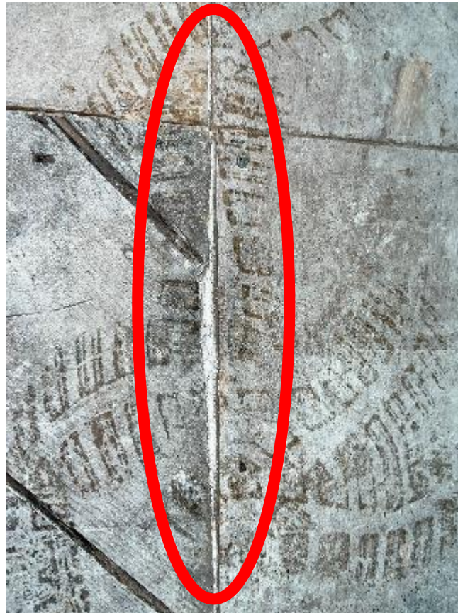
Joint in wood subfloor above basement
