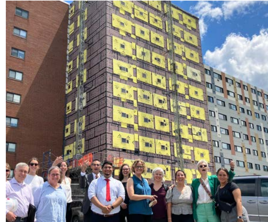
Salem Heights Deep Retrofit - POAH
