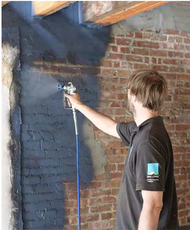
Liquid-applied air barrier
