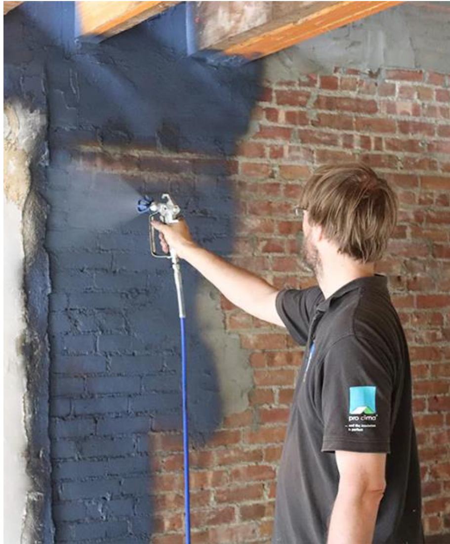
Liquid-applied air barrier
