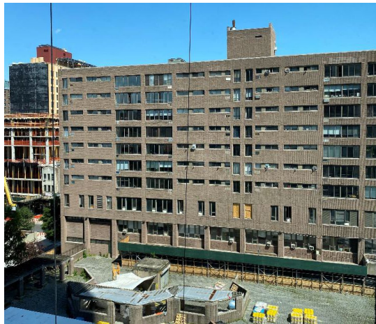
Construction staging, June 2022
