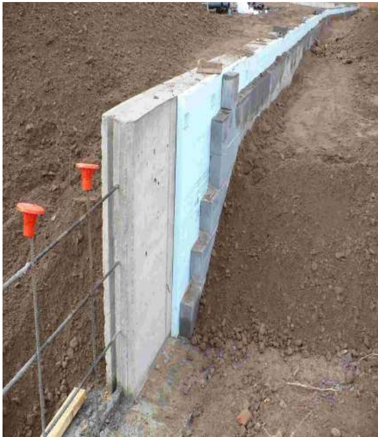
High School Classroom Addition October 2009
