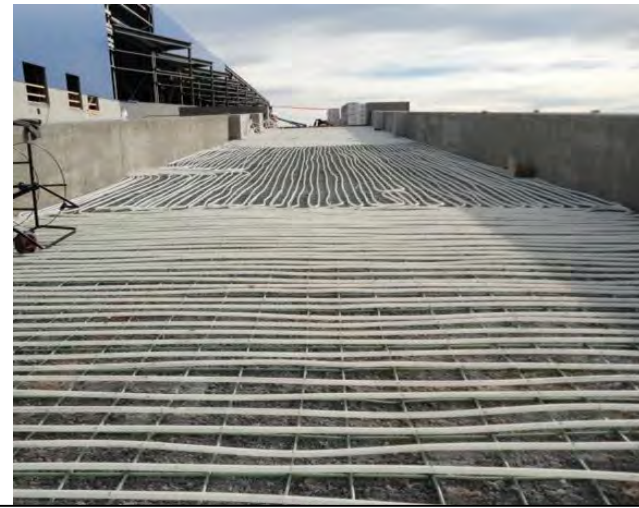
Melted Snow on Sidewalks
