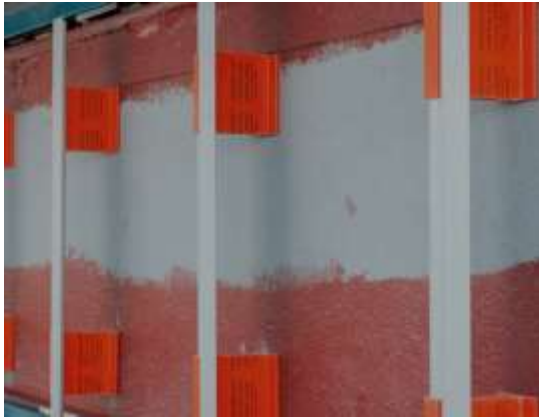
CLADDING ATTACHMENT: CASCADIA CLIPS
