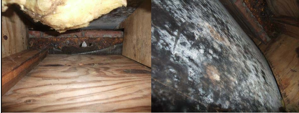
Looking upward and back towards house (wall sheathing)
