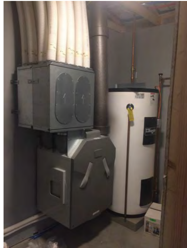
Electric water heater (Vaughn 3" polyurethane foam)
