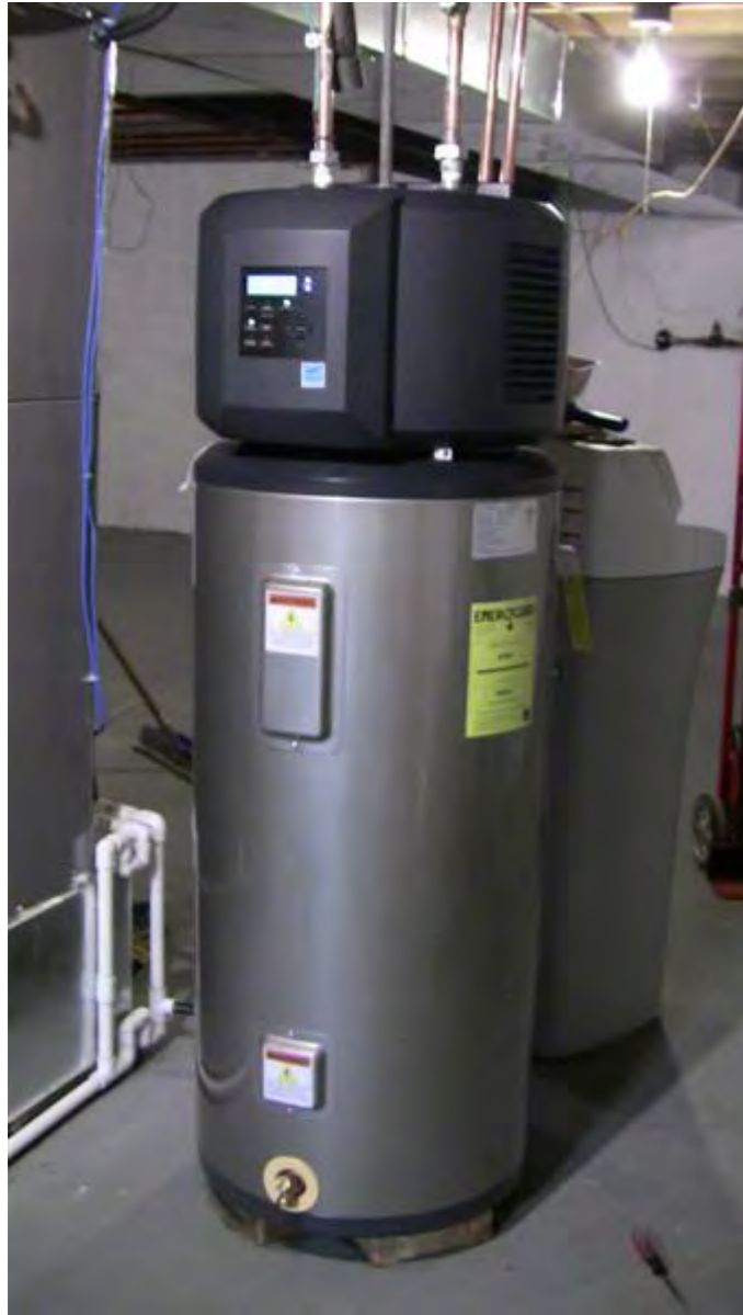
Heat Pump Water Heater
