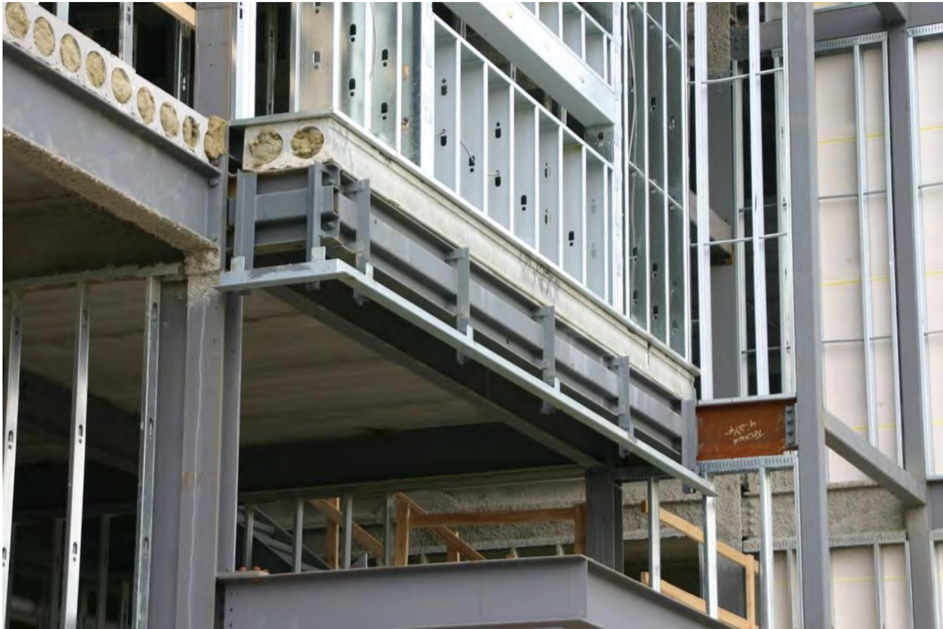
Commercial Buildings: Often exterior air barrier is the most practical solution
