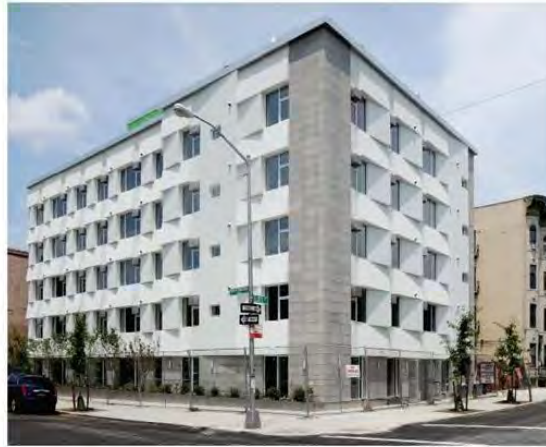
Knickerbocker Commons, the first mid-sized apartment building designed to Passive House standards in the United States
