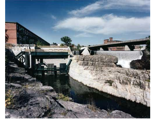
Winooski One Hydro Plant
