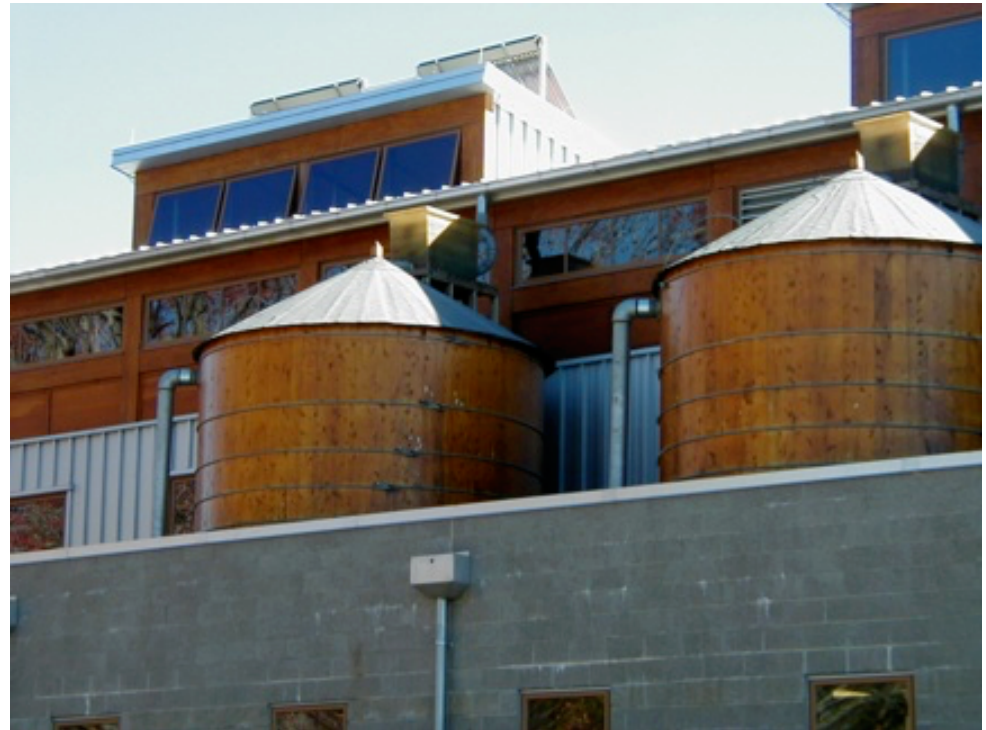
Rainwater cisterns at the Chesapeake Bay Foundation headquarters. Photo: Alex Wilson
