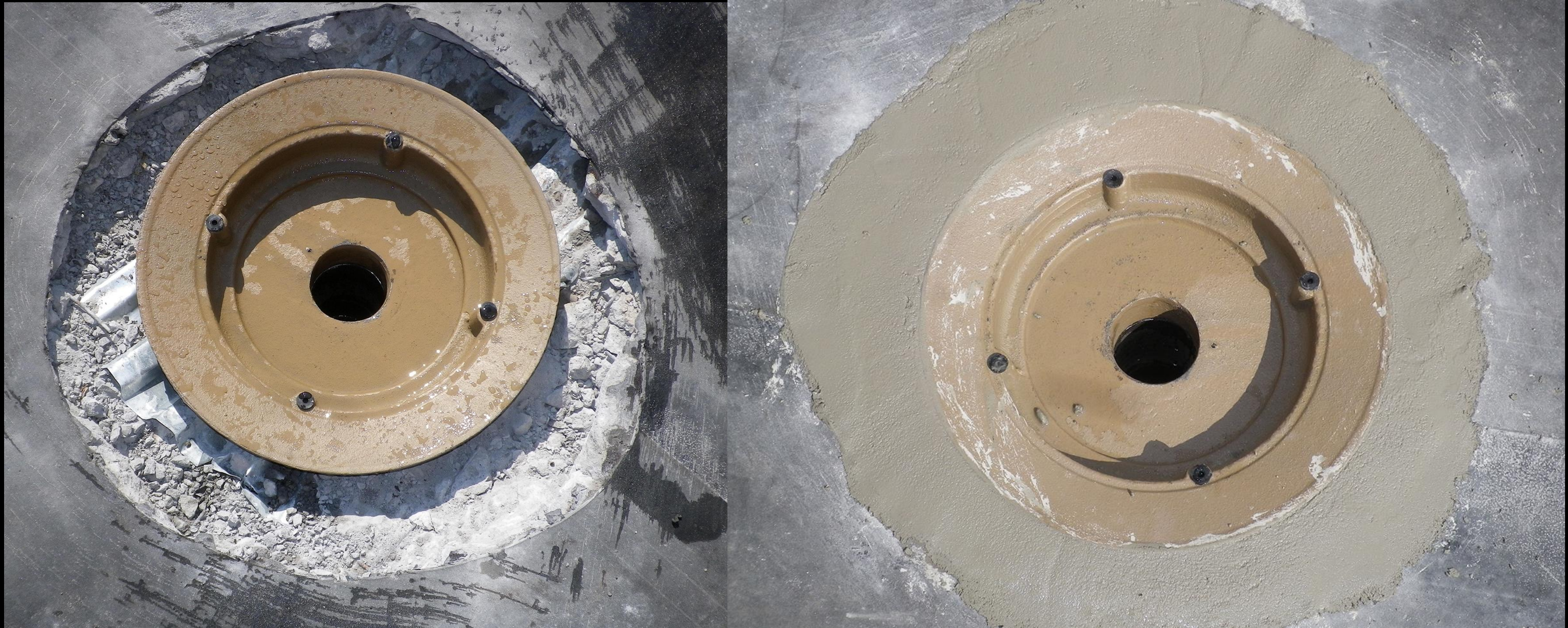
Changing the roof drains as part of a retrofit. Sensible Practice.
