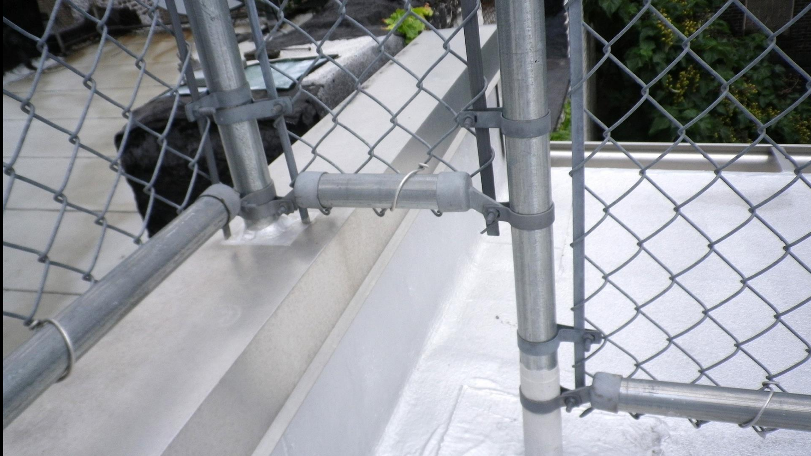
Less expensive detail. New railing posts in solid masonry. Liquid applied membrane eliminating pitch pockets.
