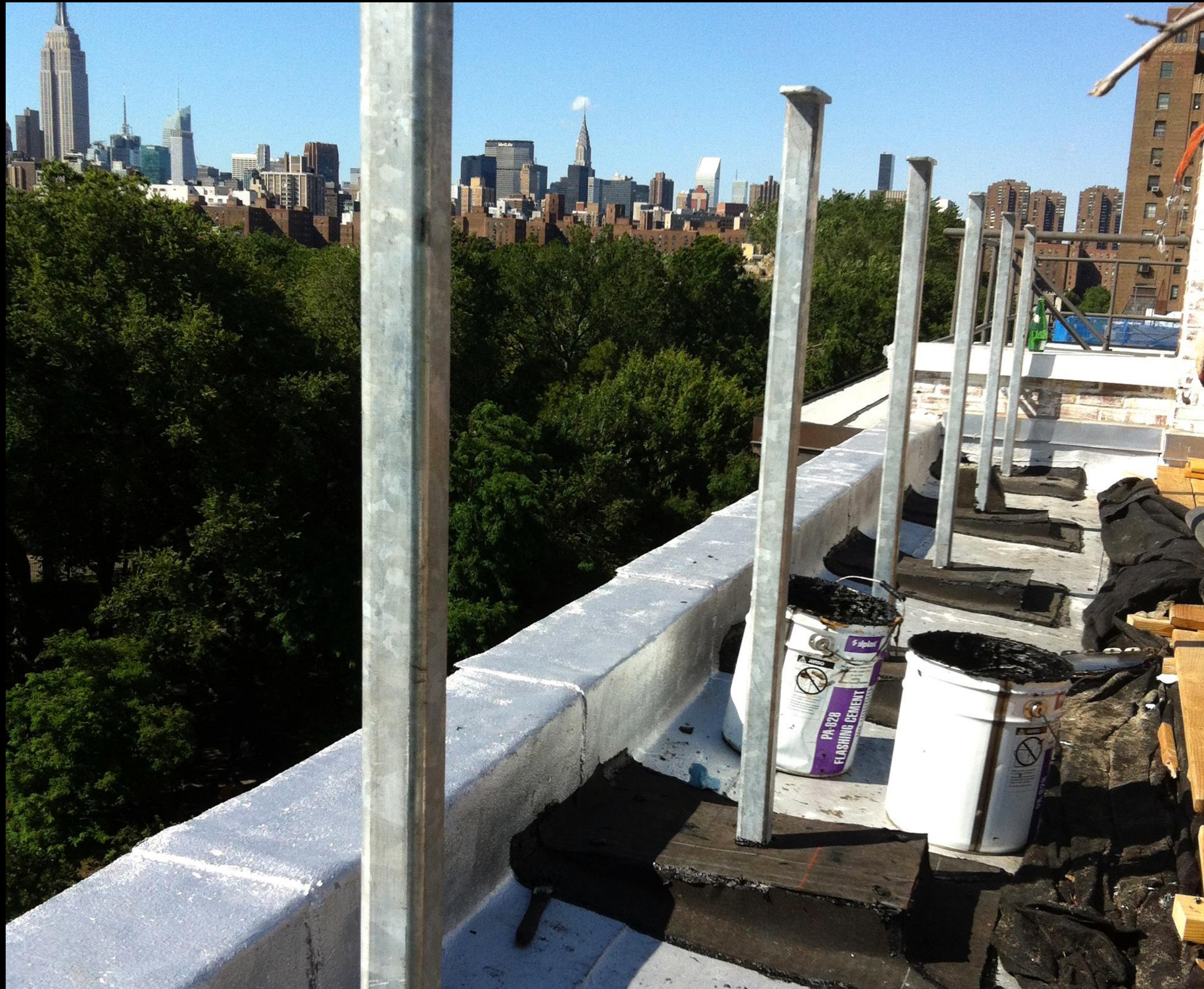
Two coats of liquid roofing applied over post base and over entire new roof membrane. Building in longevity.
