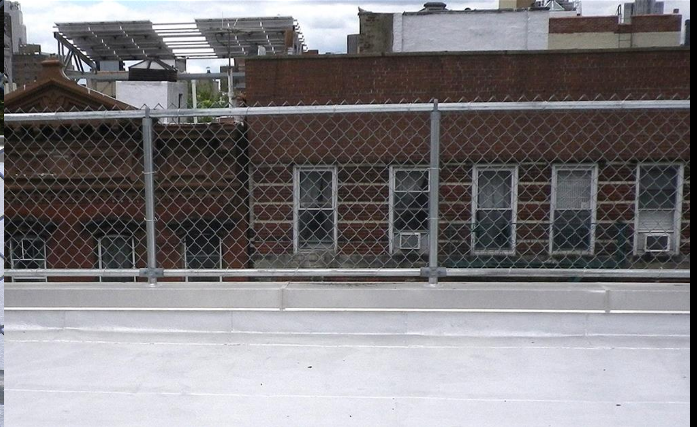
Less expensive detail. New railing posts in solid masonry. Liquid applied membrane eliminating pitch pockets.
