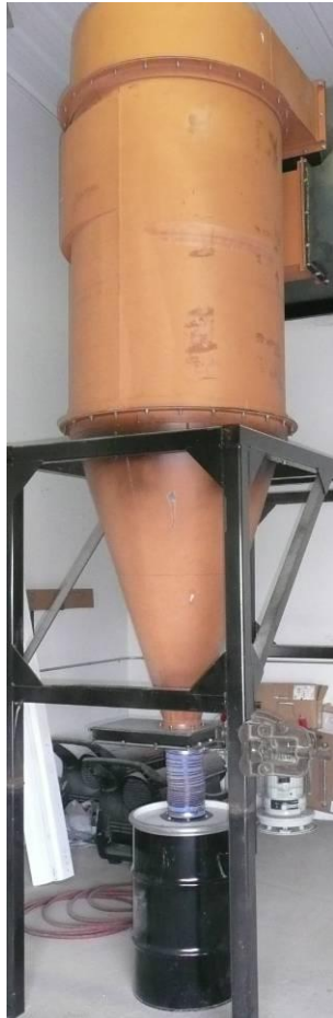
A Cyclone is often required to remove particulates from the exhaust.
